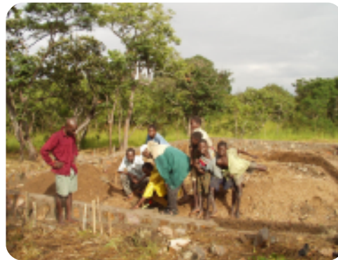
The first ground clearing for construction of the site office/engineer's house.
