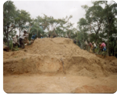
The termite mound under removal.
