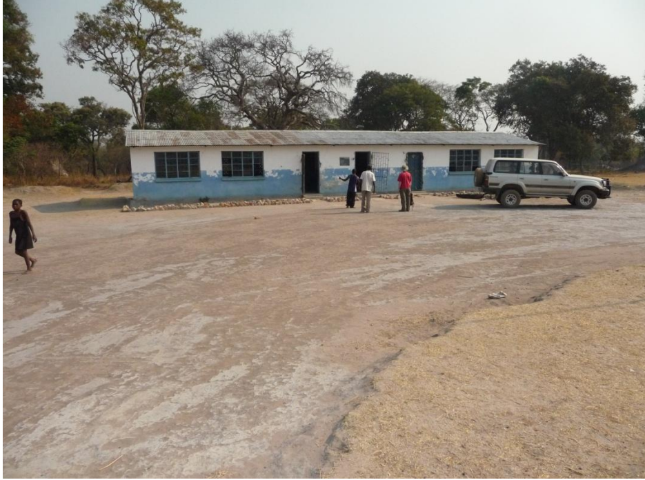
Figure 1: Single storey building with two classrooms and an office
